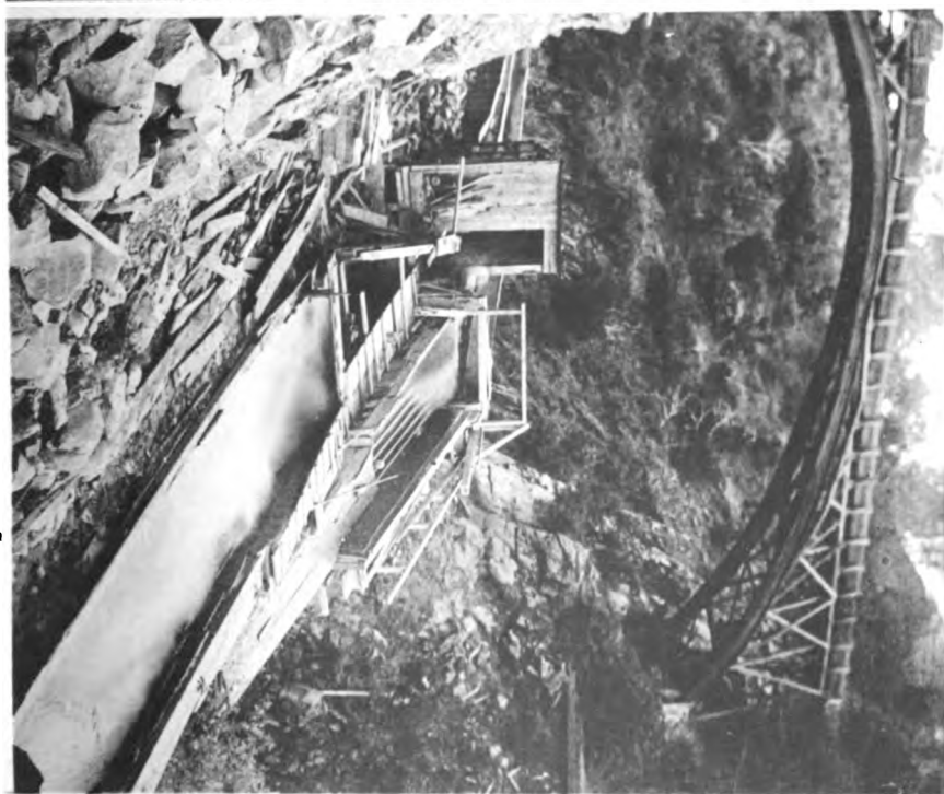
METHOD OF CARRYING FLUME ACROSS CAÑON BY IRON BRIDGE. Also grizzly for removing large boulders. Lock of room prevents introduction of undercurrent at this point.
