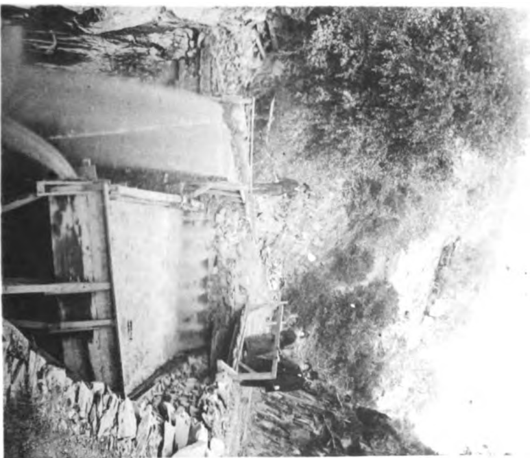
DROP FOR DISTRIBUTE GRAVEL, AND UNDERCURRENT. The material passing over the drop and that discharging from the undercurrent is taken up by sluices below.
