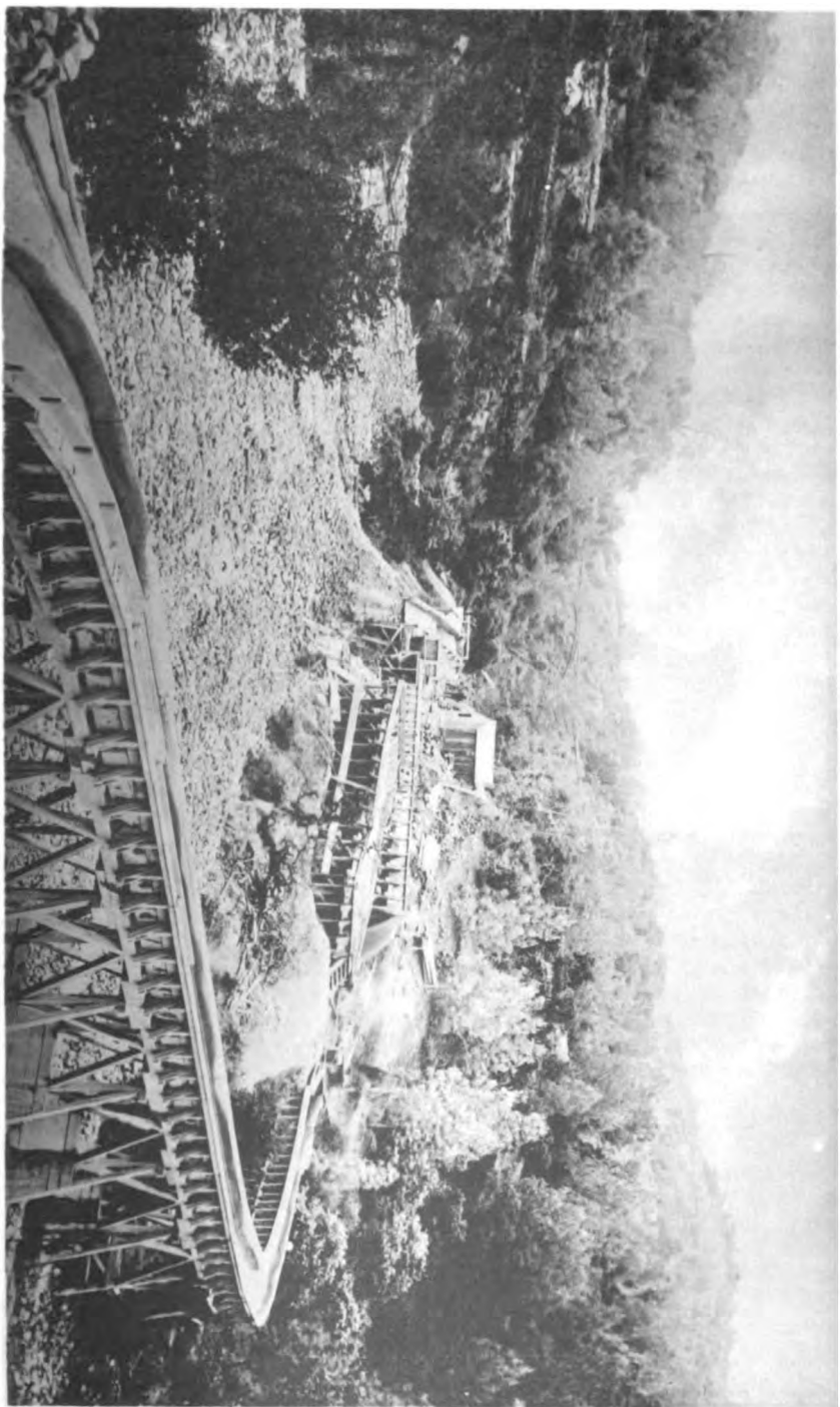
SLUICE LINE CONSTRUCTED ON CURVE.
